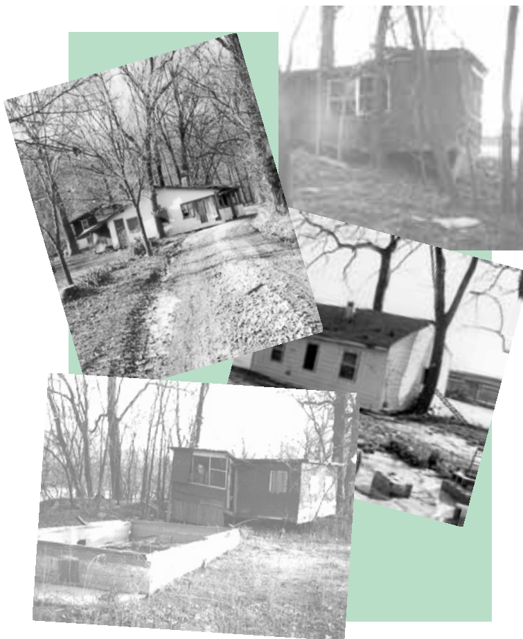
Above: Clubhouses in Fenton damaged by the 1982 flood.
