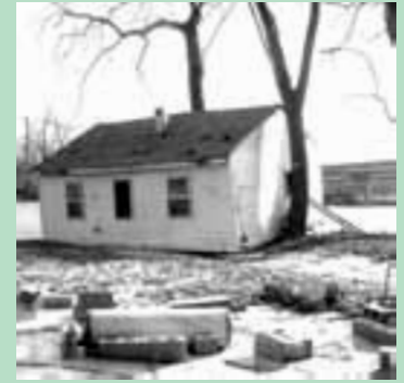
Fenton clubhouses destroyed by floods.
